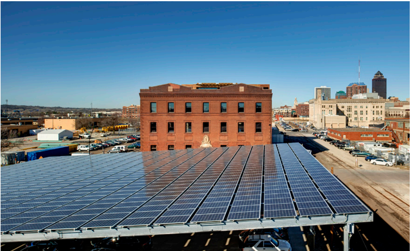
Market One—an adaptive reuse project in Des Moines—achieved LEED Platinum with over 80 points.
